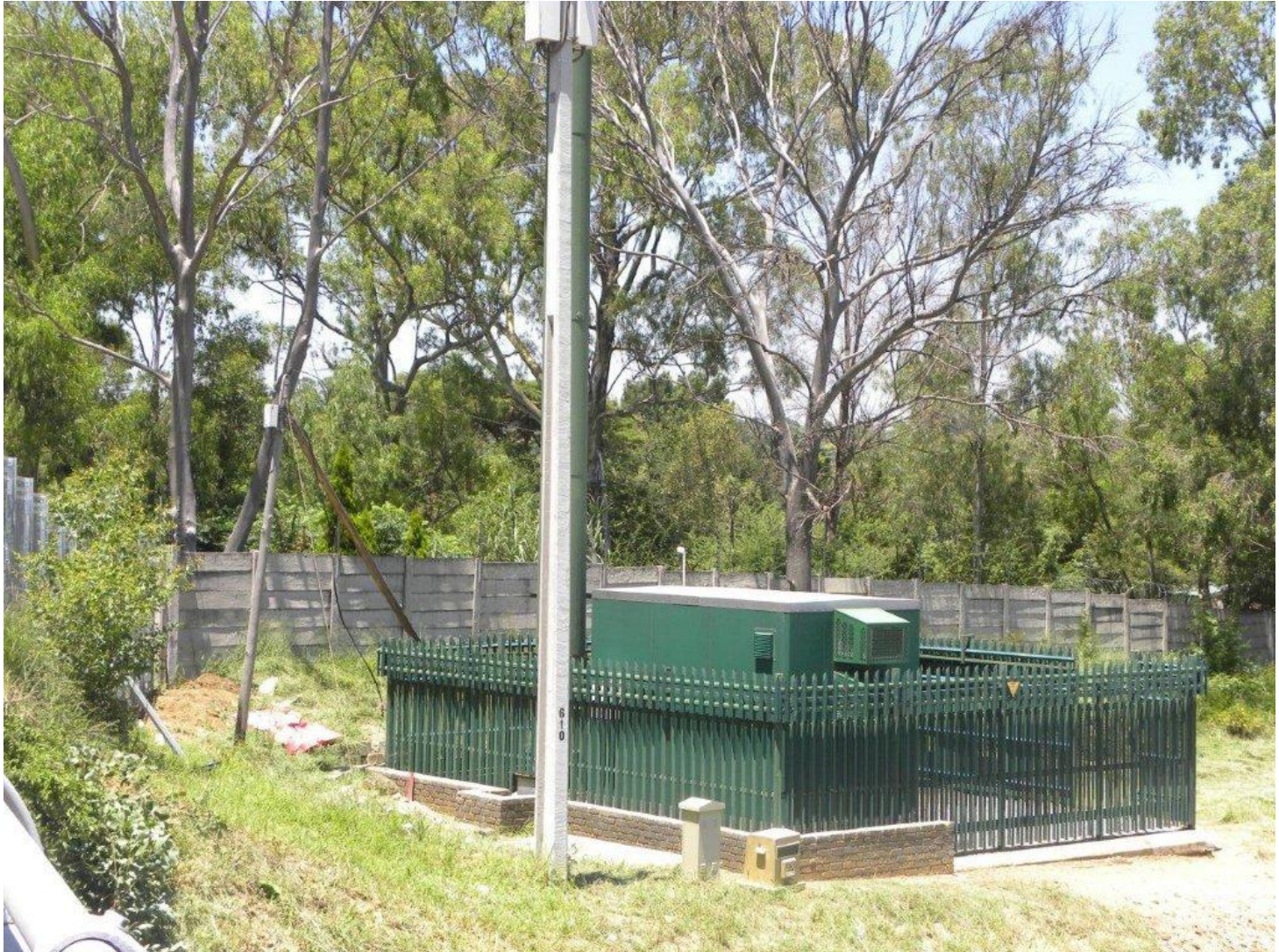
Douglas/ Grosvenor Road tower
